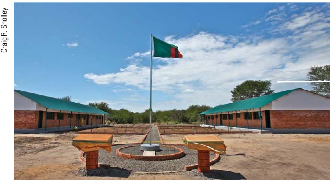
These modern classroom blocks replace an old dilapidated mud structure that was unfit for everyday use.
