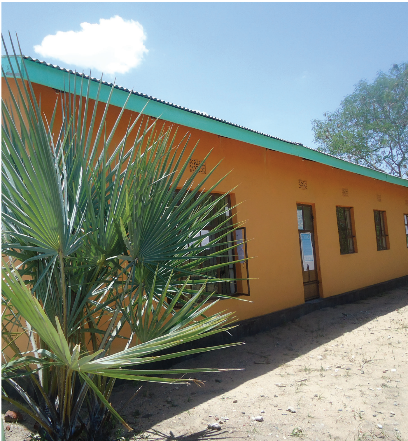
Revenues accrued from WMA, supports development projects like the construction of this village government office.
